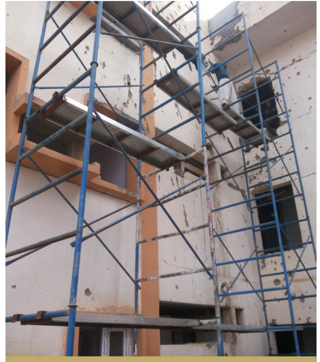
RENOVATION OF THE DOCTOR'S ACCOMMODATION WAS COMPLETED DURING THE QUARTER.
