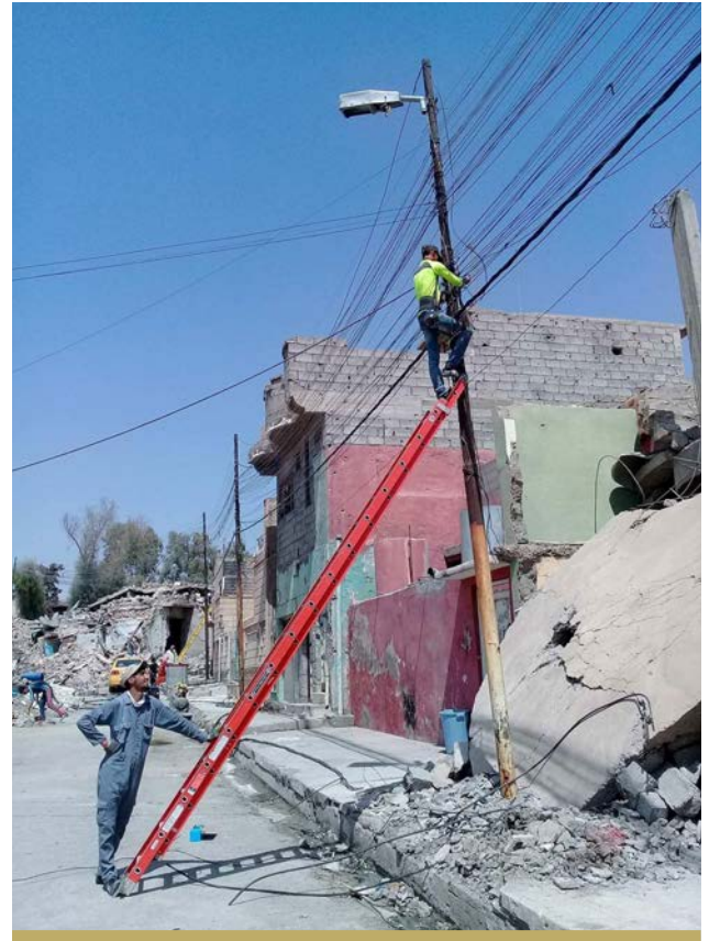
TEAMS REPAIR TRANSFORMERS IN EAST MOSUL.
