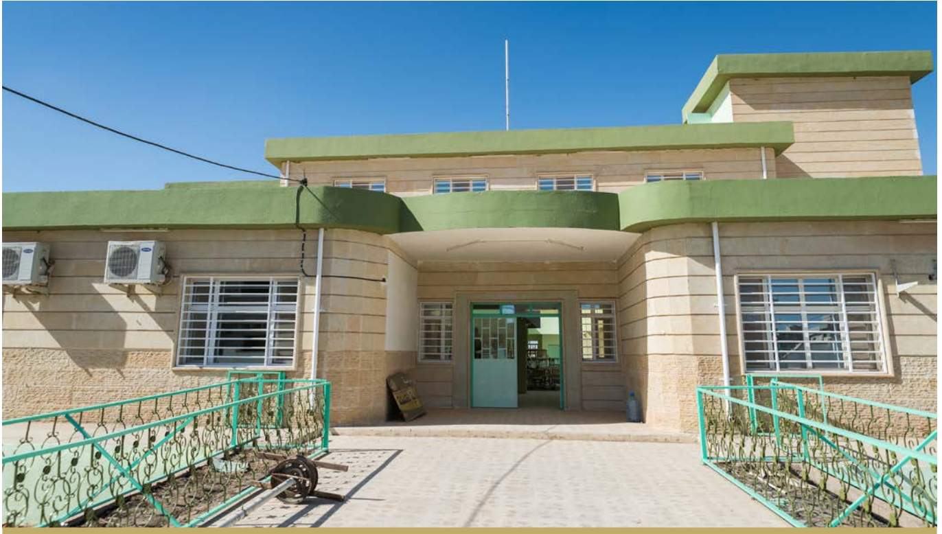
A VIEW OF THE ENTRANCE TO THE RASAN PRIMARY MIXED SCHOOL IN HAMDANIYA. THE SCHOOL WAS ONE OF DOZENS IN THE NINEWAH PLAINS UNDERGOING REPAIRS BY FFS.
